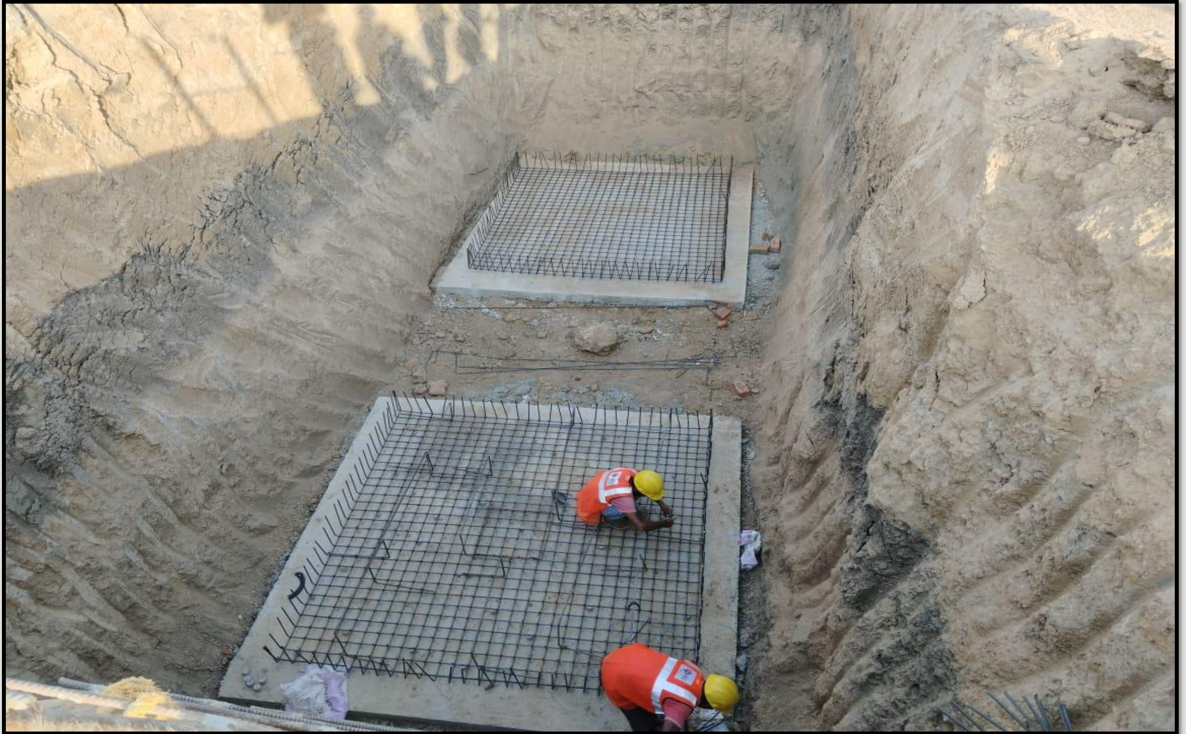
FOOTING BINDING WORK IN PROGRESS
