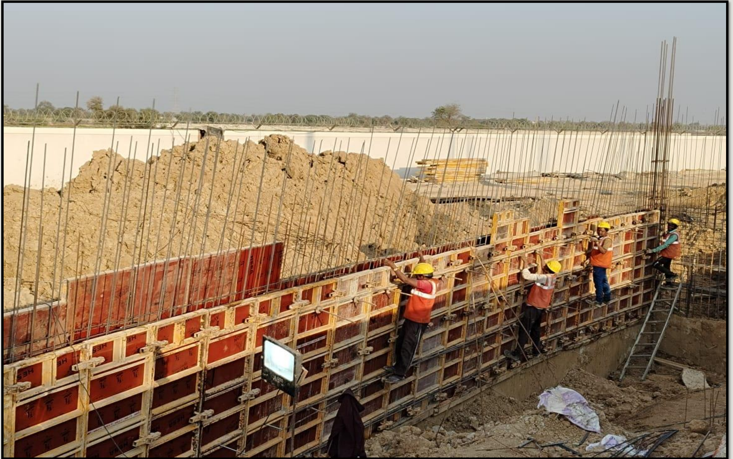
LEFT SIDE RAMP WALL SHUTTERING WORK IN PROGRESS.
